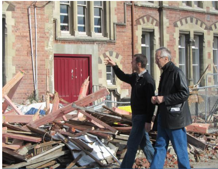
Christchurch, New Zealand, February 25, 2011 -- Tim Manning, left, Deputy Administrator for Protection and National Preparedness at the Federal Emergency Management Agency, inspecting earthquake damage in Christchurch. Manning was in Christchurch attending a U.S.-N.Z. Partnership Forum when the earthquake struck. FEMA/U.S. Embassy-New Zealand/Janine Burns
